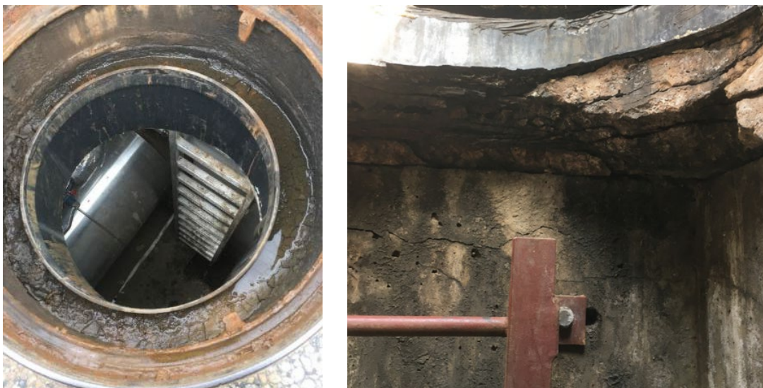
Figure 5.12. Inspection of DH network chambers (photo by Öresundskraft AB)
