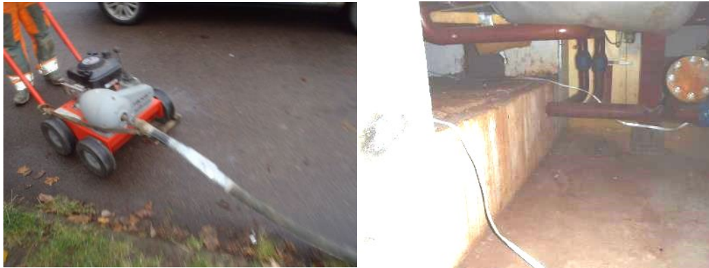
Figure 4.9. Electric tapes laid down in the impassable reinforced concrete channel
