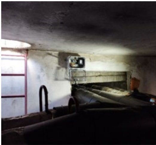
Figure 5.4. Sensor station on the DH grid (OPEC, Wejherowo) (photo by Gdańsk University of Technology)
