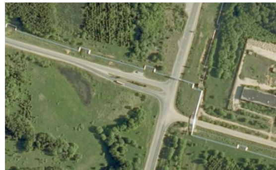
16 km length overland pipeline built from the former Ignalina nuclear power plant to the city of Visaginas, Lithuanian
