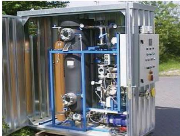
Figure 4.22. Mobile helium (He) injection plant (by AGFW)
