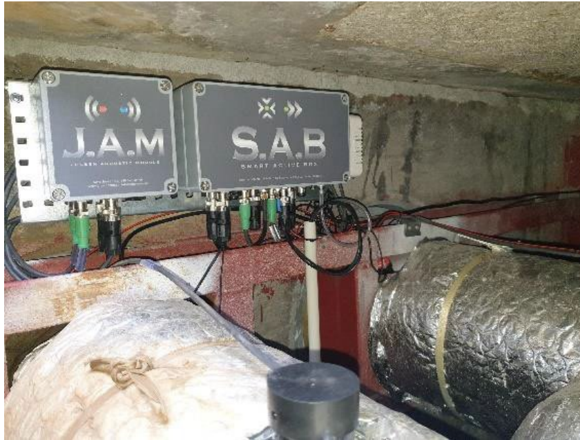
Figure 5.11. Arrangement of devices for measurement of tube wall thickness in the DH chamber (photo by Öresundskraft)
