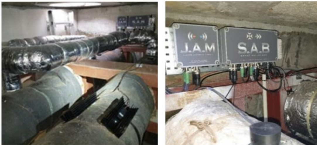
Figure 4.29. The SAB condition monitoring system (data from SweHeat and Öresundskraft)
