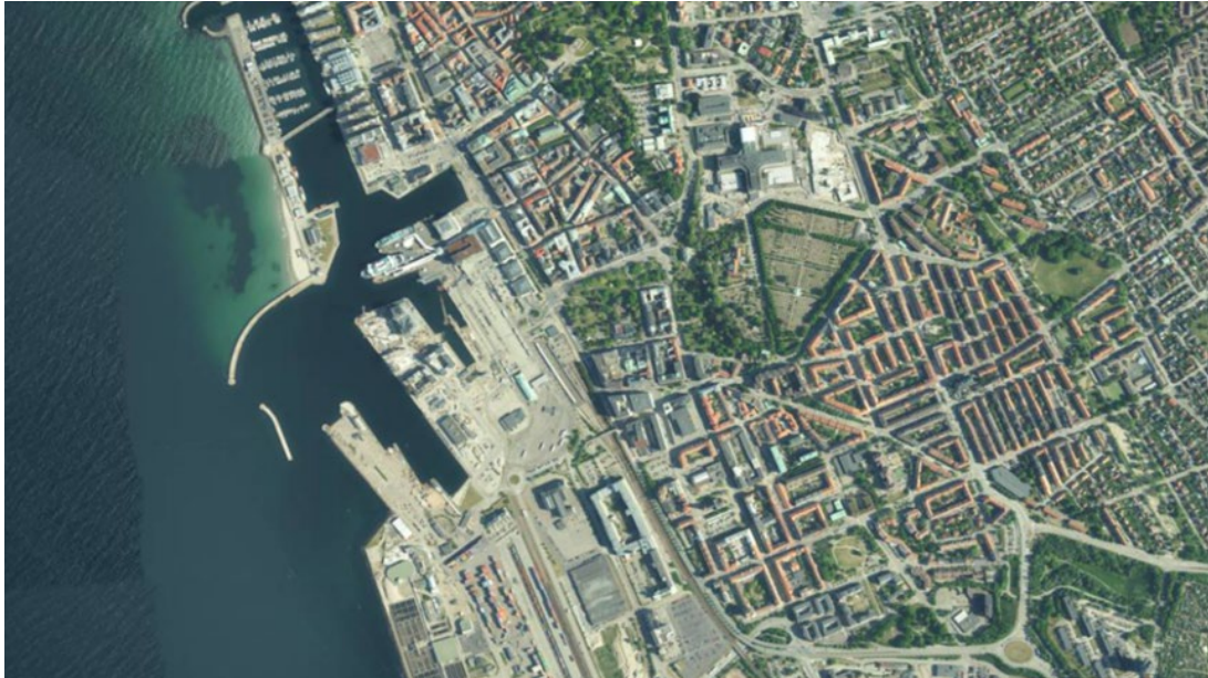
Figure 5.10. Furutorpsgatan in Helsingborg with 500 m of concrete culvert chosen for a pilot case of 10 chambers (photo by Öresundskraft)
