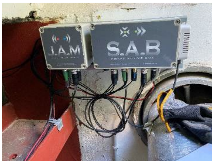
Figure 1. Installation of SAB in a chamber
