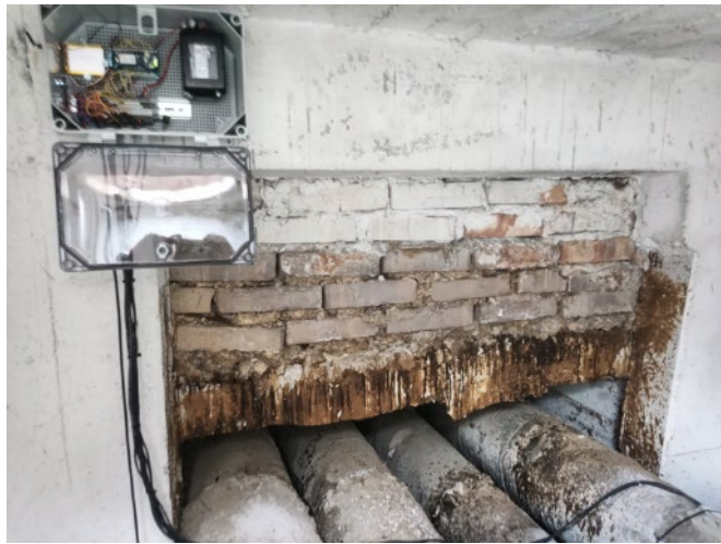
Figure 5.3. Installation of sensor stations in Wejherowo (OPEC DH grid) (photo by Gdańsk University of Technology)
