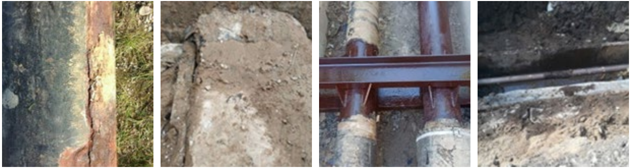
Poor waterproofing
